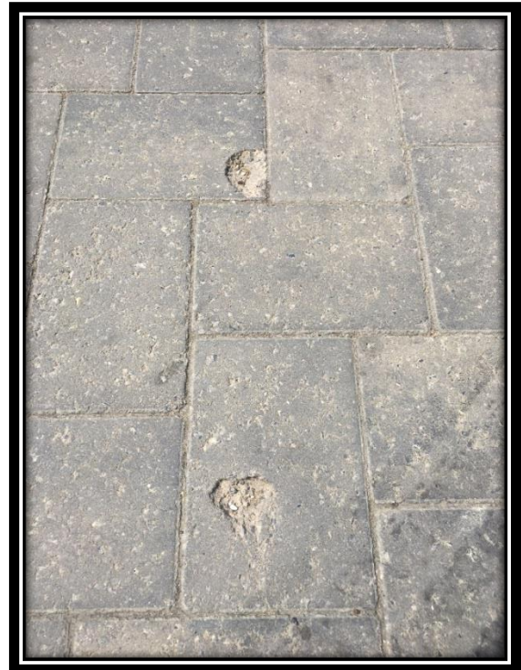
Damage to Block Paved Roads – Example 2
